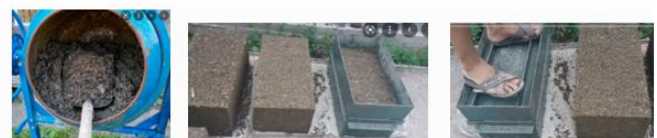
Figure 3. The preparation of arbolit briquettes [3].
