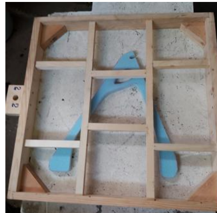
Fig.2. Made in advance special casting boxes
